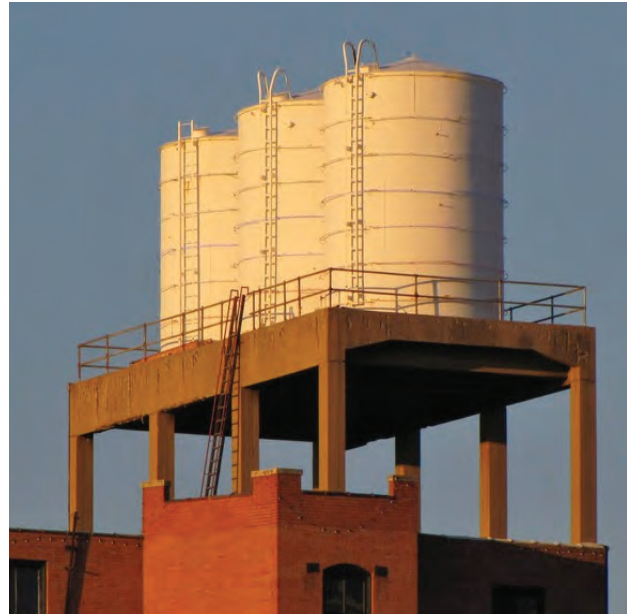
Overhead water tanks
