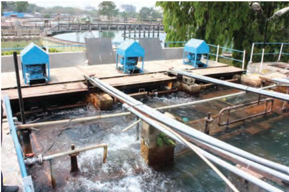
**Oxygenation :** Air and water are allowed to mix with the help of pumps. This causes oxygen from the air to dissolve in the water.
