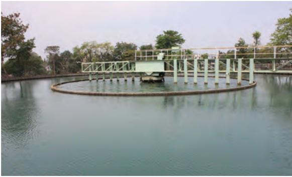
**Settling-** The water from the water source is allowed to stand in large tanks. Alum is also used to help the process of settling.
