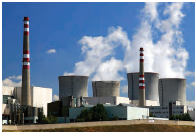
Figure 9.17 : An Atomic Power Generation Plant
