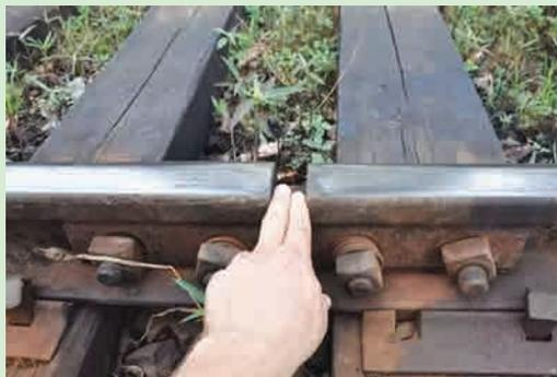
Similar to rails, the length of bridges can also increase due to expansion in summer. The length of the 18 km long great belt bridge in Denmark increases by 4.7 m in summer. Therefore, provision is made in the construction of the bridges to accommodate this expansion.
