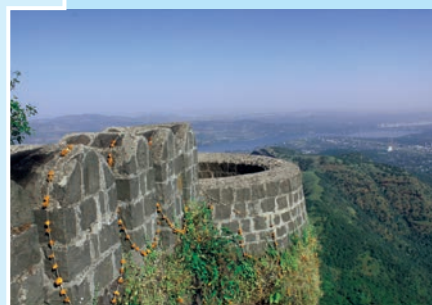
Figure 1.13 : Khadakwasla Dam as seen from Sinhagad
