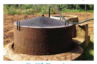
Fig. 10.7: Biogas plant
