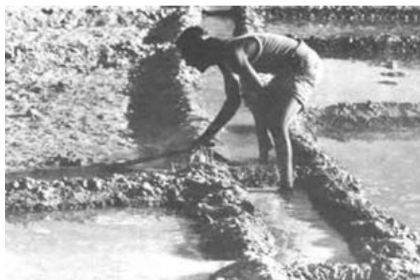
Fig 7.2 : Check Basin method
