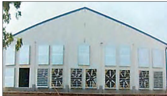
House with exhaust fans
