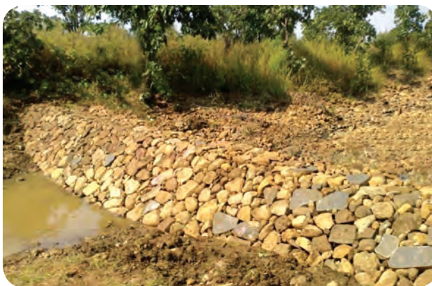
Fig. 6.11 : Loose rock check dam
