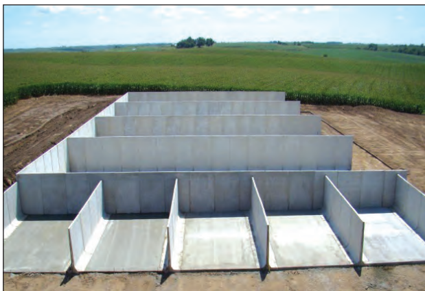
Fig. 8.5 Horizontal trench silo
