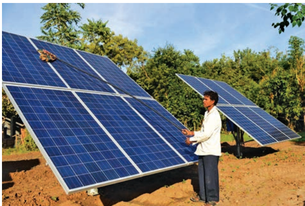
Solar panels - Non-Conventional Energy Source
