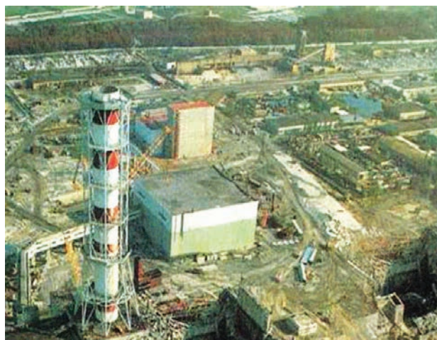
Chernobyl nuclear power plant after the explosion
